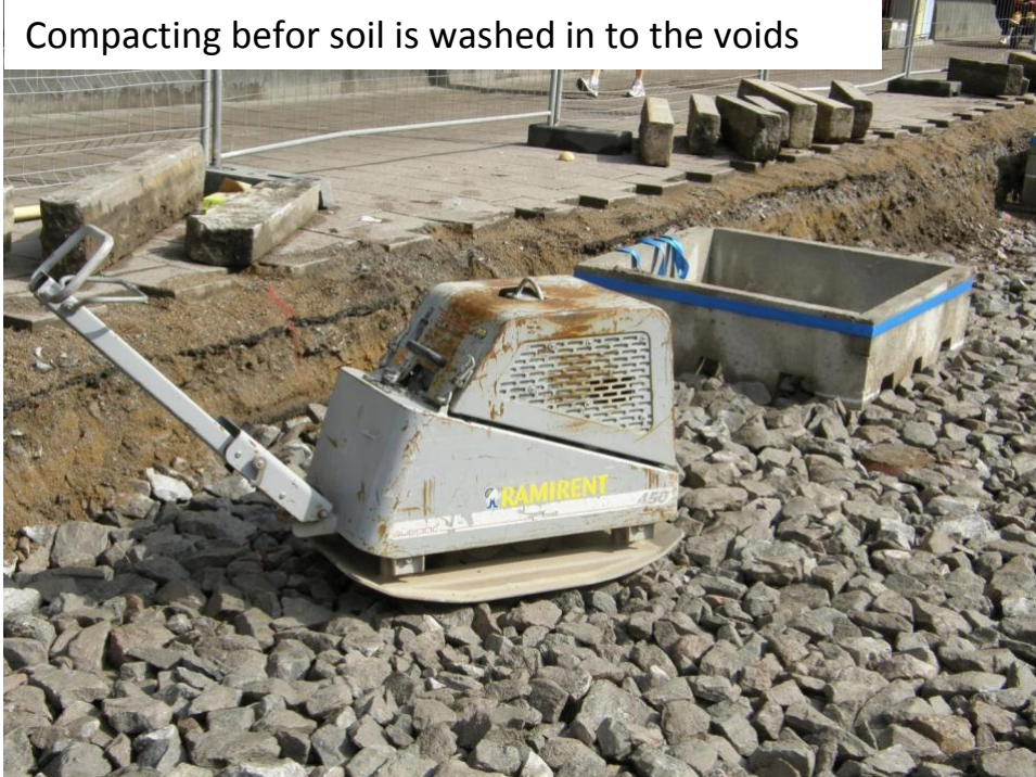
The stone shall fall into the box to get a stable construction
