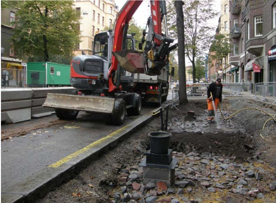
Flushing the soil into the structure
