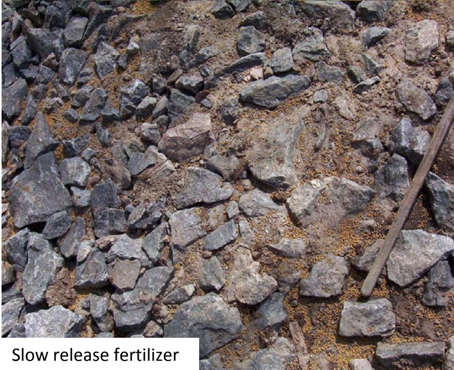
Layer for infiltration of surface water and aeration of the soil on top off the structural soil
