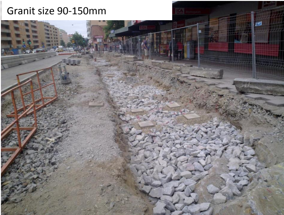
Compacting befor soil is washed in to the voids
