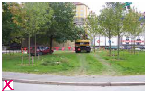
No cordon around the trees: The setup of this project site allows cars and heavy machinery to repeatedly compact soil in the root zone of these trees, and drive through the crowns as well.
