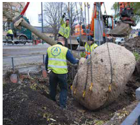
The root ball on a tree with a stem girth of 60-70 cm.
