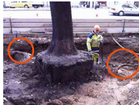
Pipeline roots exposed during excavation.
