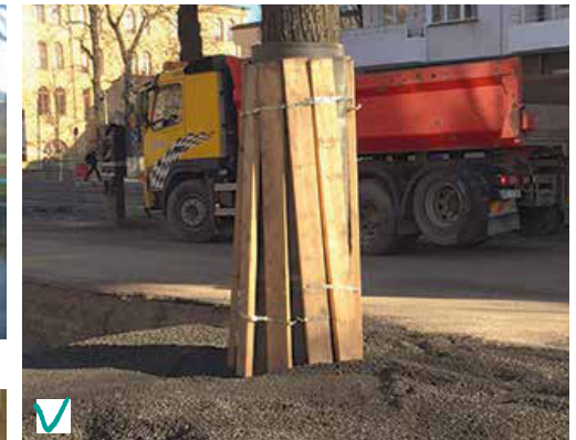
Trees protected with cover and boards for plant bed renovation. Photo Lovisa Hell.
