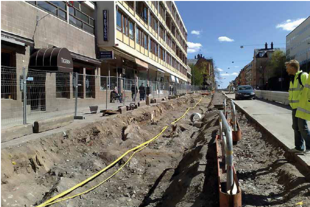
What is in the ground – rock, gravel, sand or clay?
