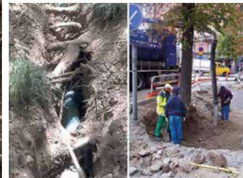
Tunneling of pipe under roots using vacuum excavation.
