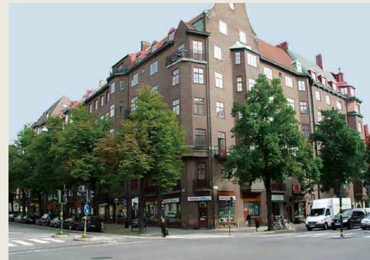
The existing trees on the right have been given new plant beds – Birger Jarlsgatan.
