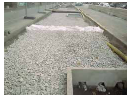
The geotextile dam in aerated bearing layer.
