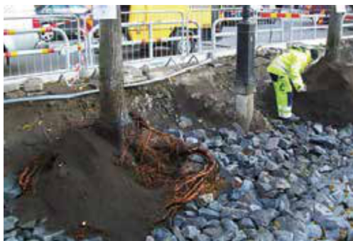
Plant bed renovation on Birger Jarlsgatan.
