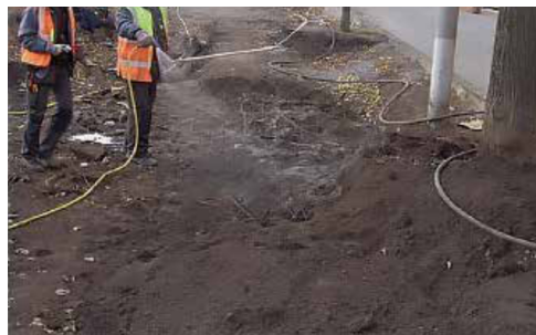
Irrigation of exposed roots.
